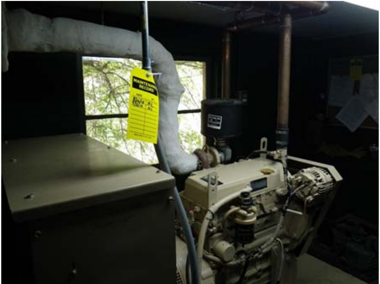
Informational Photo No. 3: Interior of Woonsocket Falls Dam showing existing window to be replaced.
