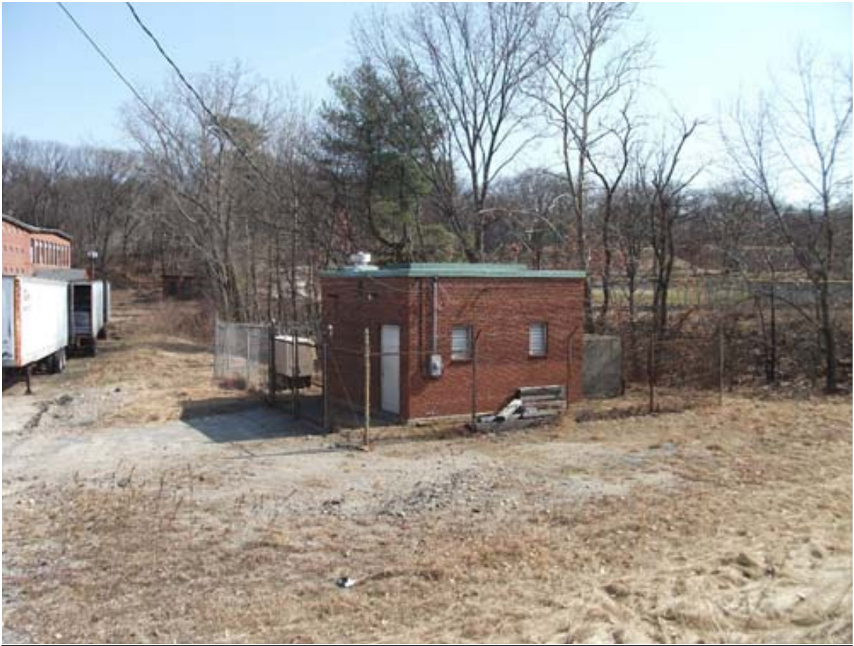
Informational Photo No. 1: Singleton Street Pumping Station, view of exterior door and two of four vents to be replaced with top hinged windows.
