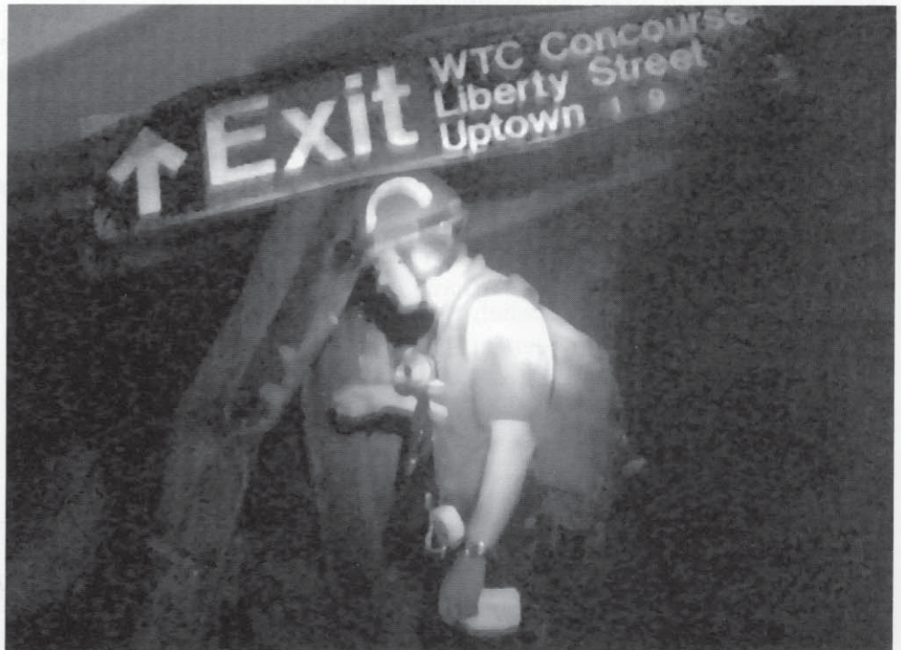
Mark Wingate, a structural engineer from San Francisco District on a severely damaged subway platform under what used to be the World Trade Center station stop.
