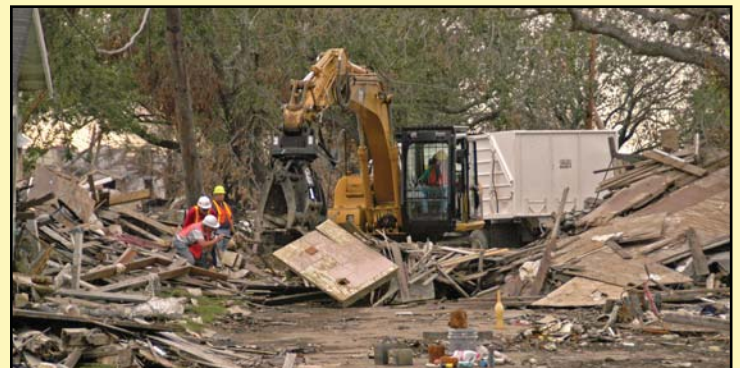
Corps of Engineers debris management specialists check debris being cleared in New Orleans for hazards and/or human remains after Hurricane Katrina in 2005. The Corps' largest debris mission came after the 2005 hurricane season, when more than 72 million cubic yards of debris was removed from multiple Gulf Coast states following the hurricanes that battered the region. (Photo by Marvin Nauman, FEMA)
