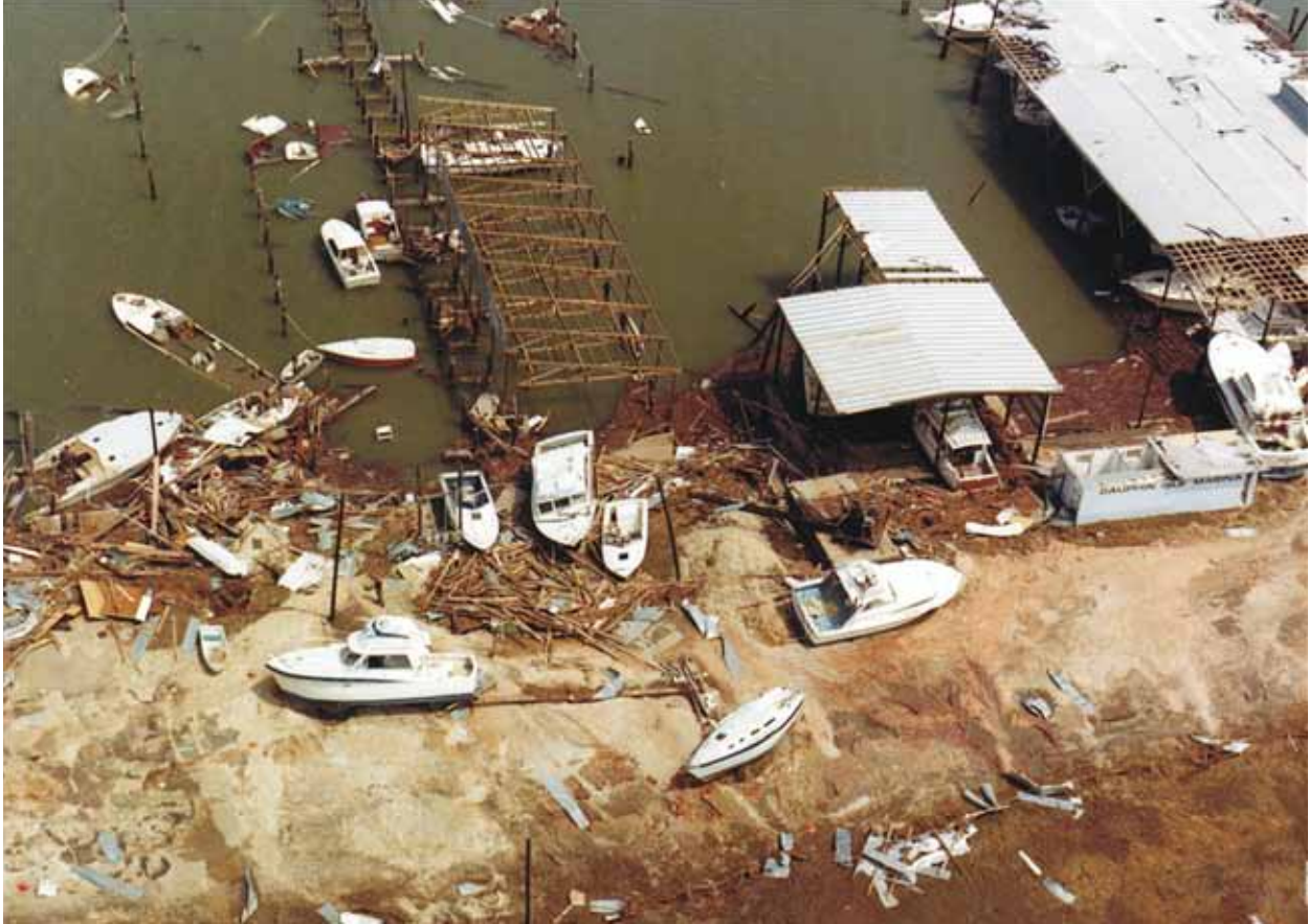
Damage on Dauphin Island from Hurricane Frederick 1979.
