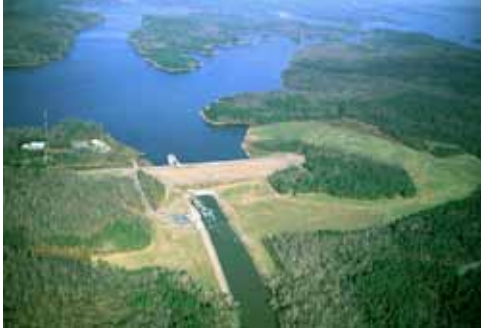
The Jordan Dam on the New Hope River, North Carolina.
