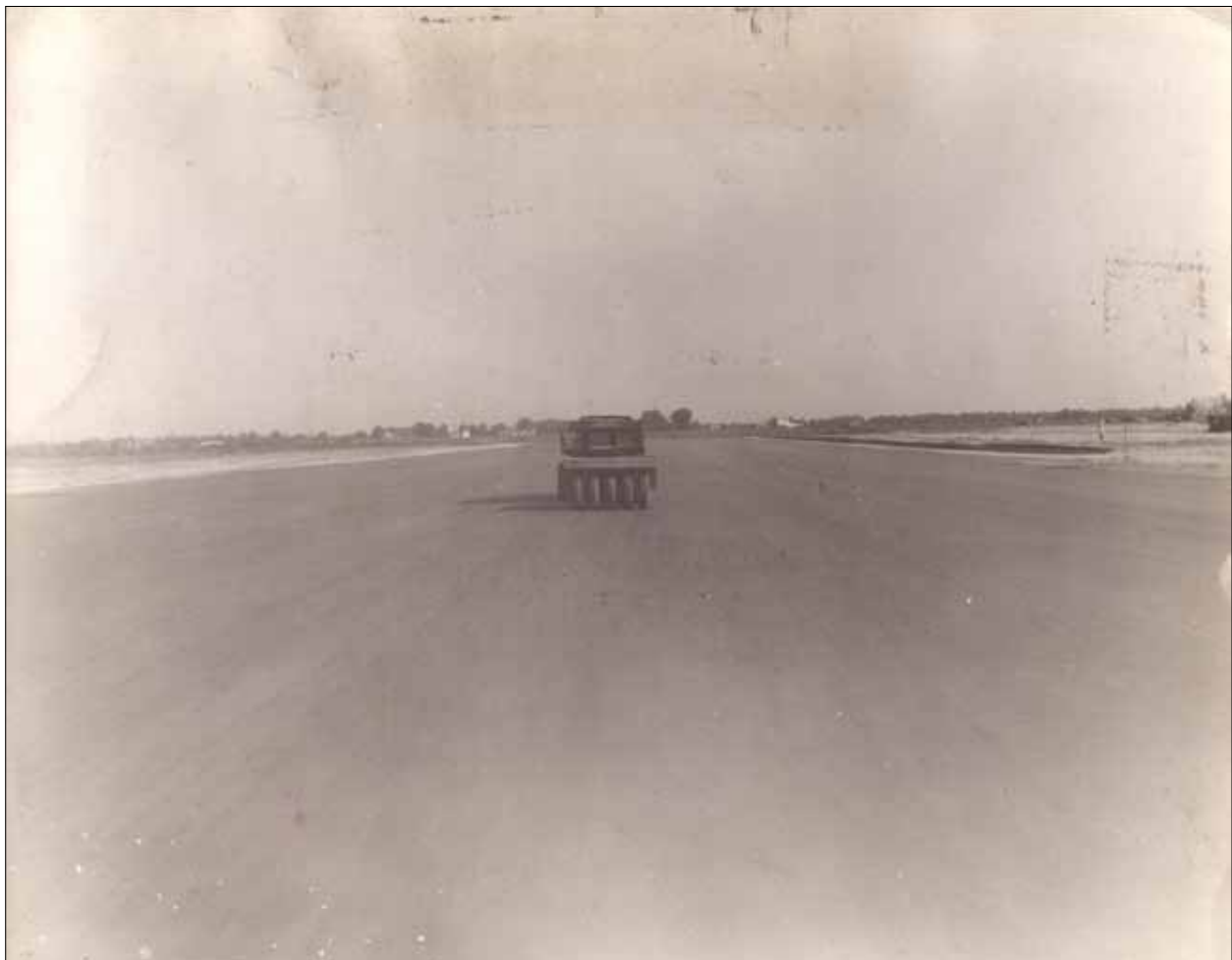
CAA Florence Municipal Airport Under Construction, Florence, S.C. (USACE photo).
