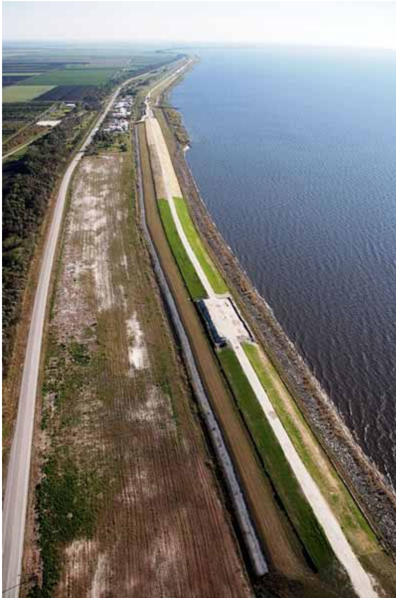
The Herbert Hoover Dike surrounding Lake Okeechobee in Florida was identified as high risk for structural failure in a study following the Hurricane Katrina disaster.
