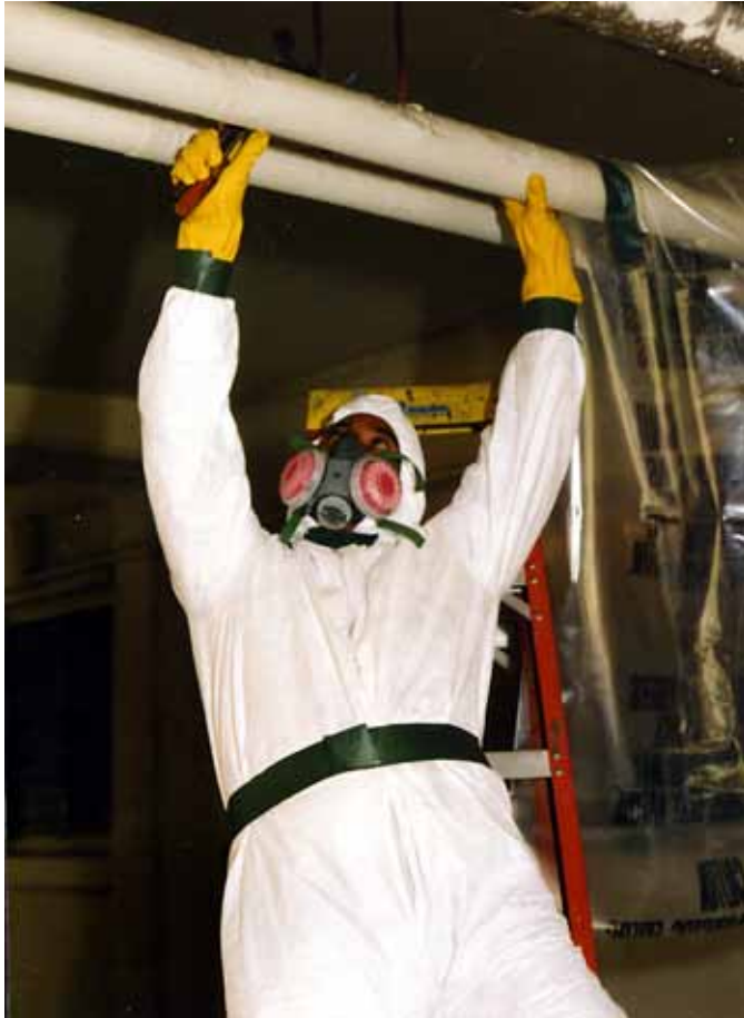
Corps employees remove asbestos at Canal Zone structures.
