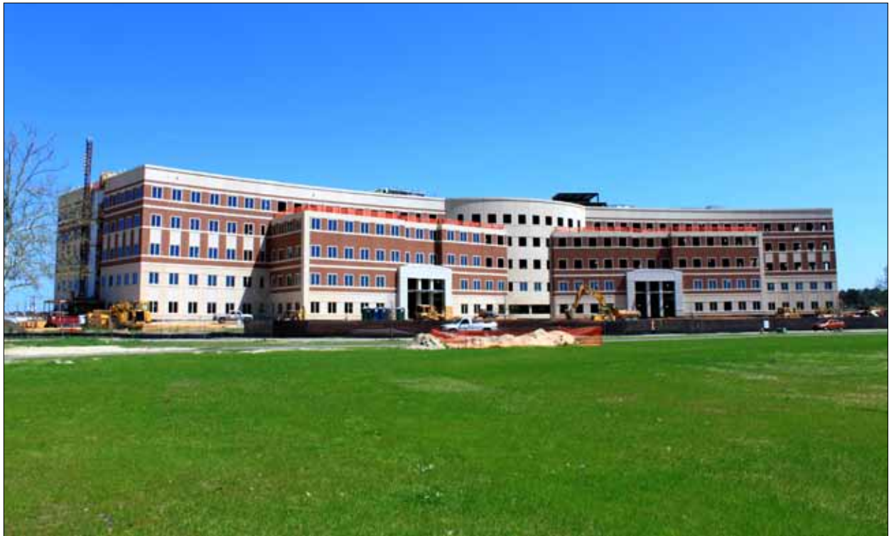
The new joint FORSCOM-USARC headquarters building at Fort Bragg, North Carolina opened for business in 2011.
