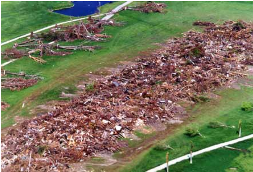
Damage in Homestead from Hurricane Andrew. Photo taken several days after the storm.
