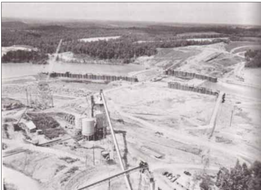
Hartwell Dam under construction, 1958.
