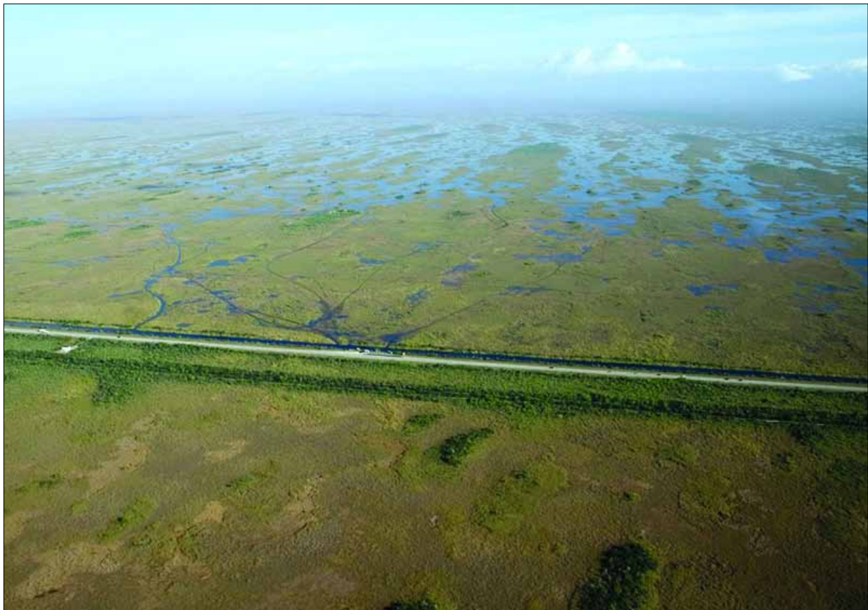
The Tamiami Trail, officially designated US 41, stretches 264 miles across south Florida between Tampa and Miami. While offering beautiful vistas of the Everglades, the raised roadway disrupts the natural water sheet flow feeding delicate natural habitats.
