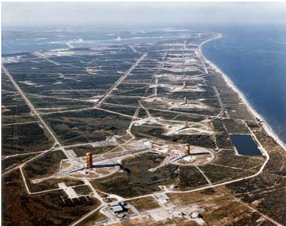
Aerial view of Missile Row, Cape Canaveral Air Force Station, looking north.
