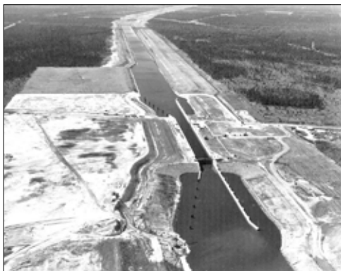
A completed section of the Cross Florida Barge Canal, excavated through dry land.
