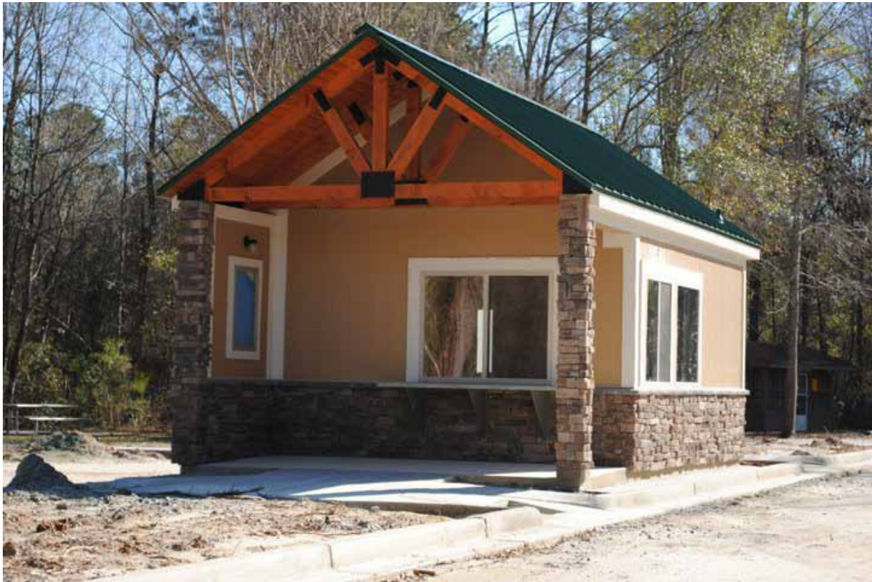
Even the smallest ARRA project made a difference. This restroom at Lake Walter F. George is now ADA compliant.
