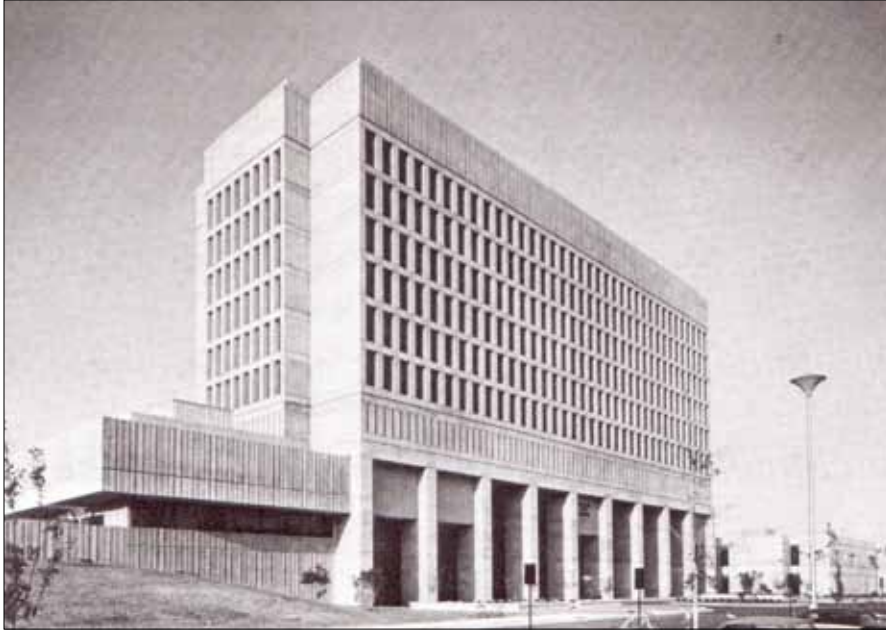
Moncrief Hospital at Fort Jackson, S.C. (Savannah District).
