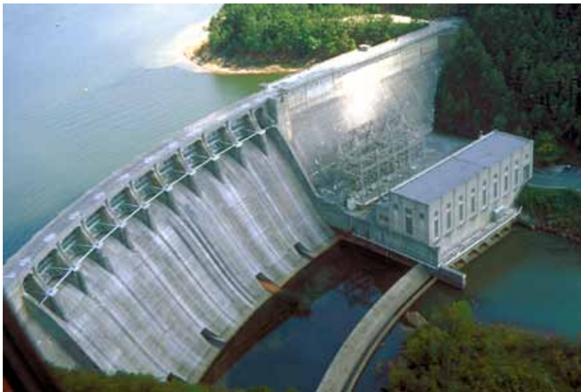
Allatoona Dam and Lake north of Atlanta, Georgia was one of the first reservoir projects after World War II (USACE photo).
