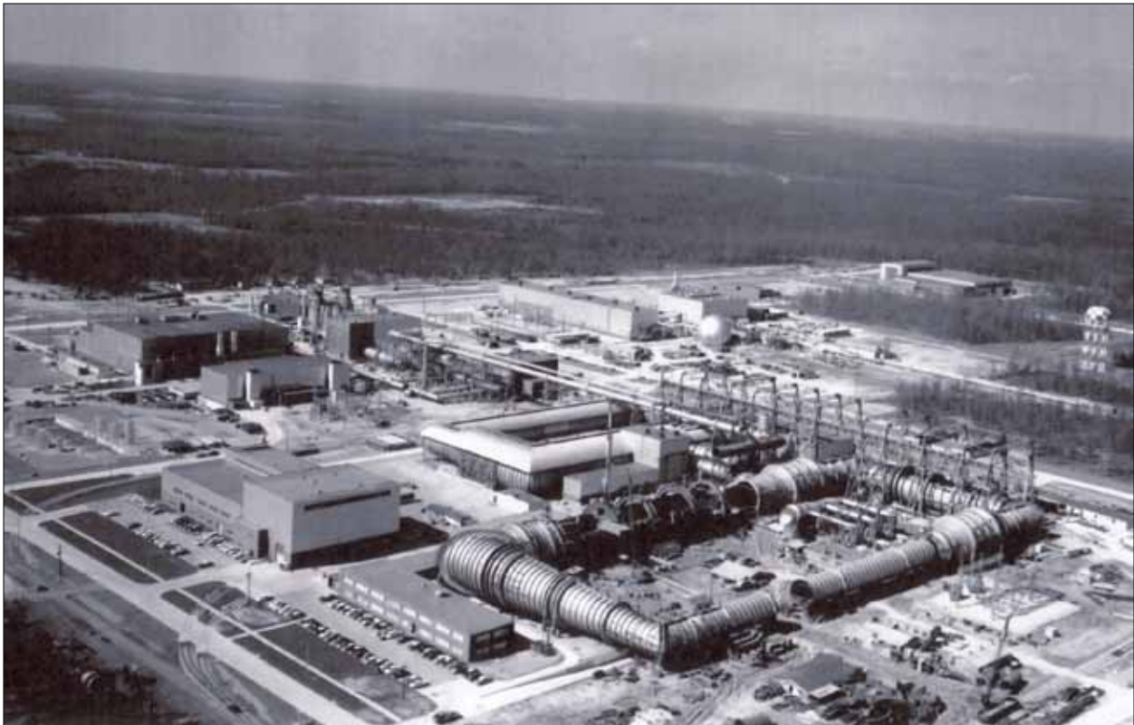
Arnold Engineering Development Center, 1958 (USACE photo).
