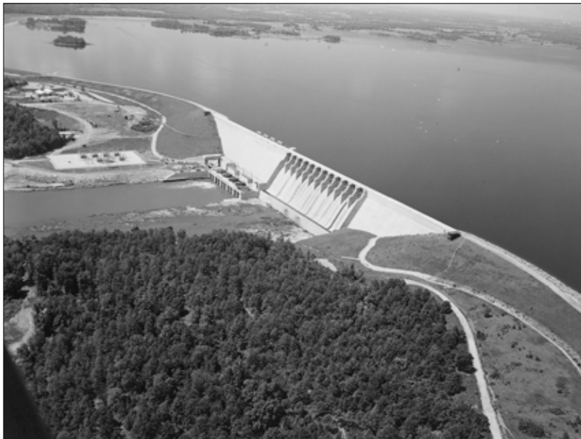
The Hartwell Dam and Reservoir was the first of three large multipurpose projects completed by SAD districts in the post-World War II period on the Savannah River (USACE photo).
