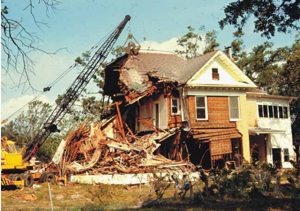
Corps contractors take down a destroyed house after Hurricane Camille.
