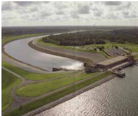
The St. Stephen powerhouse in the Cooper River Rediversion Canal.
