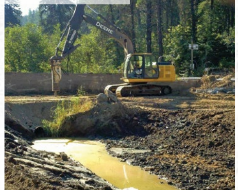
Photo 9. Removal of the Dutch Flat Dam
