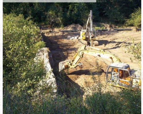
Photo 8. Exposing the back side of Dutch Flat Dam
