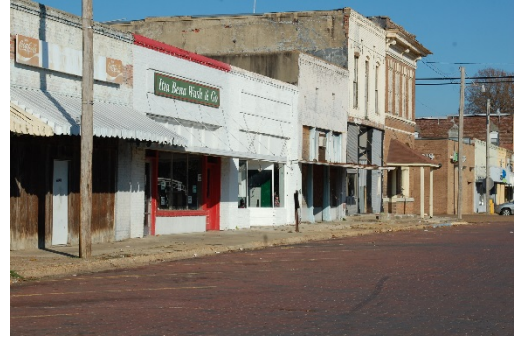
Itta Bena's downtown is a mixture of local businesses and vacant buildings in need of revitalization and reuse (Source: Connie Perkins)
