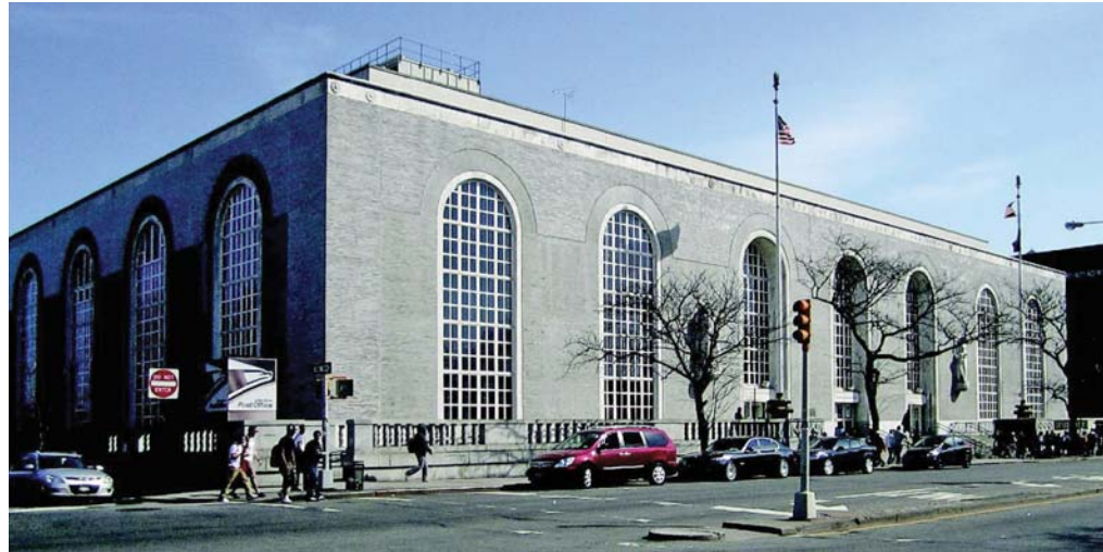
» BRONX, NEW YORK COLONIAL REVIVAL, 1936 Credit: USPS
