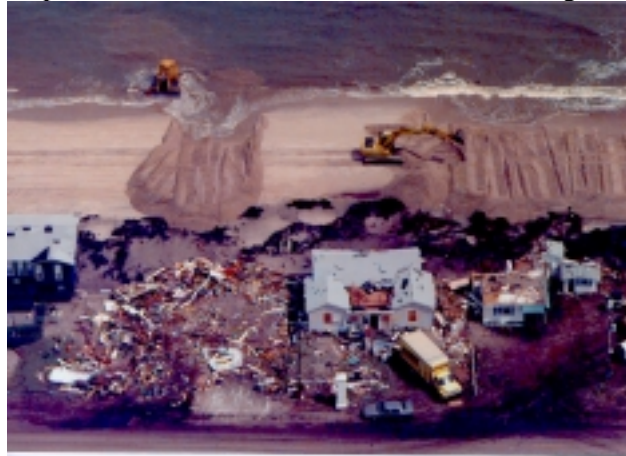
FIGURE 4.7 After oceanfront homes at Kure Beach, North Carolina, were destroyed by Hurricane Fran, attempts were made in 1996 to rebuild dunes along the coast.
