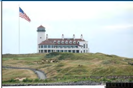
Bayonne Landfill: 4MCY (+ many other landfills & Brownfields remediated)
