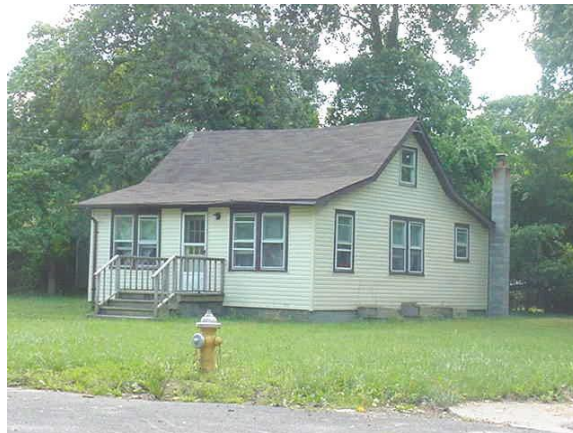
Figure 3: Typical Raised (Crawlspace) Foundation Type
