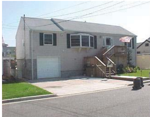
Figure 6: Typical Raised Ranch Structure Type
