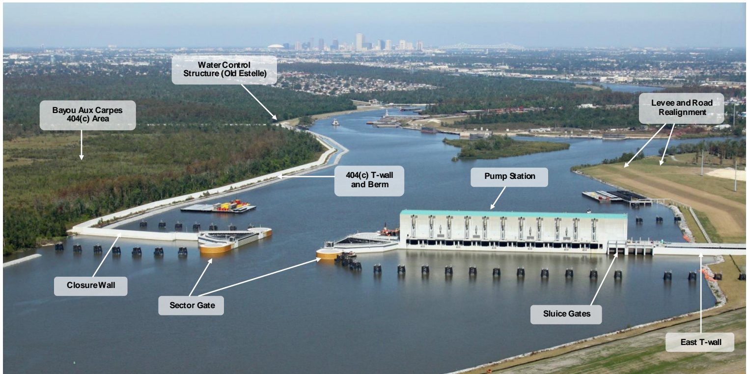
Image of the GIWW-West Closure Complex
