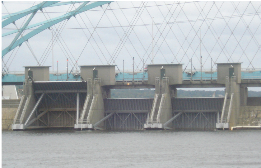
Fox Point Hurricane Barrier in Providence, Rhode Island.
