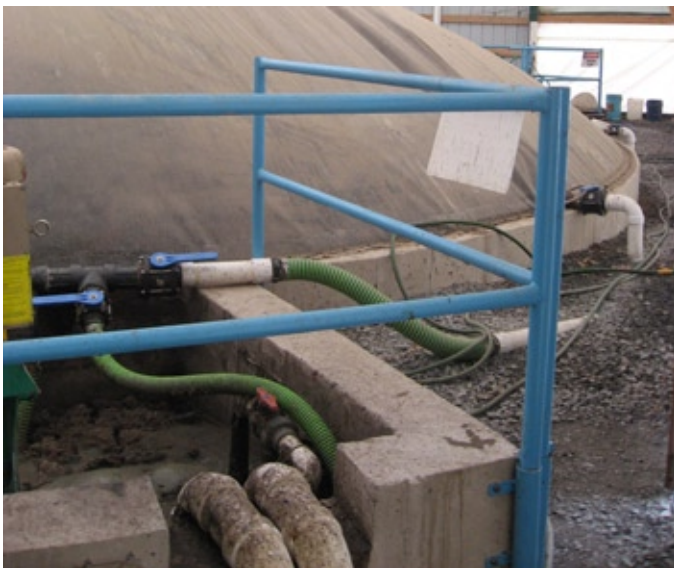
Digester inlet pit
