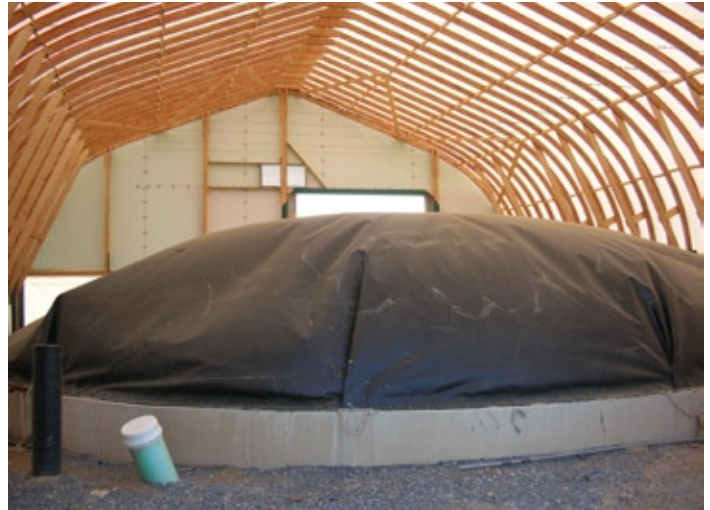
Wood framed arch building over the digester
