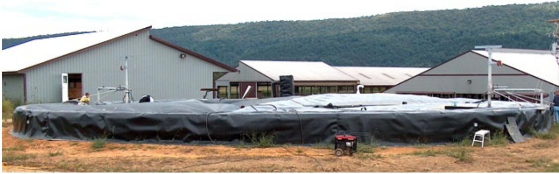
Digester with flat cover
