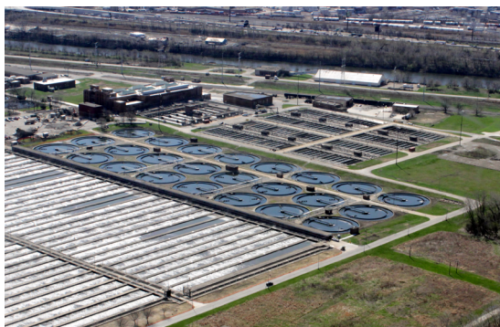
Aerial view of Stickney Wastewater Treatment Plant. US Army Corps of Engineers photo.
