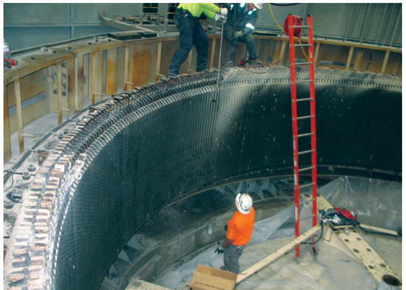
Alstom Power technicians remove winding coil halves from the stator core of Carters Reversible Pump Turbine Generator 4. At a contract cost of nearly $20 million, authorized by GA-AL-SC System customers, the electrical components of two versatile and drought critical generators will be replaced. Photo:USACE
