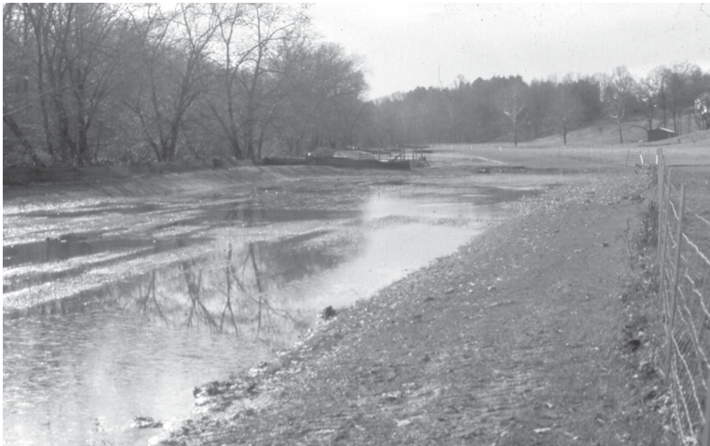
Figure 12-2.—A riparian created wetland made by excavating upland soils down to the presumed winter high water table. This site receives considerable surface and ground water inputs. Excavation of more than 30 in (0.75 m) of soil was required with considerable soil disturbance and compaction. (Photo courtesy of Steve Long, Virginia Department of Transportation. )
