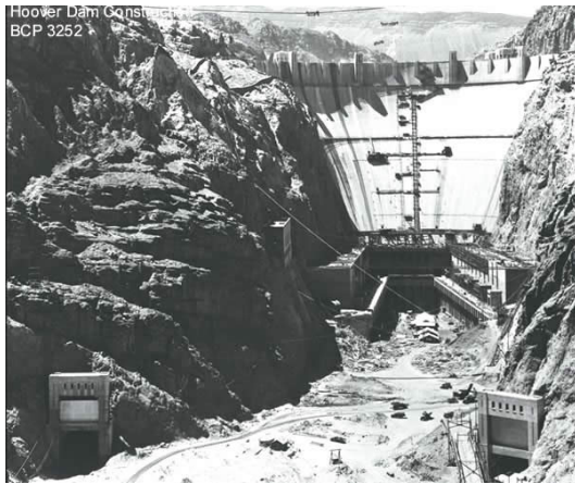
Boulder Dam During Construction
