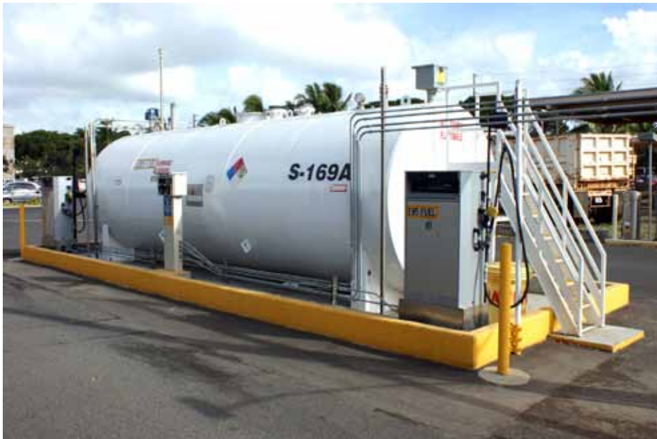
PEARL HARBOR (March 22, 2012) The U.S. Navy has opened the first E85 station at Joint Base Pearl Harbor-Hickam. The 10,000-gallon tank contains 85 percent plant-based ethanol blended with 15 percent gasoline which can be used in all flex-fuel vehicles. Two more Navy E85 stations are planned to open. Marine Corps Base, Hawaii has the only other E85 station in the state. U.S. Navy photo by Denise Emley.
