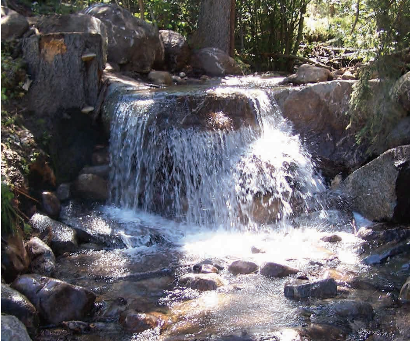
Constructed fish barrier to protect a population of Rio Grande Cutthroat trout. USFWS Photo.
