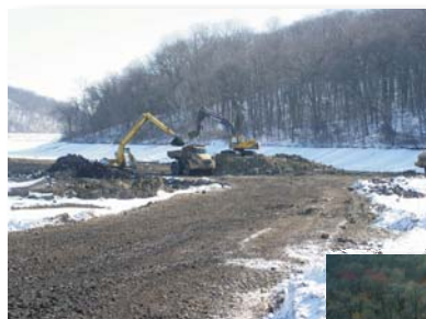
Sediment removal from behind the dam. Winter 2003
