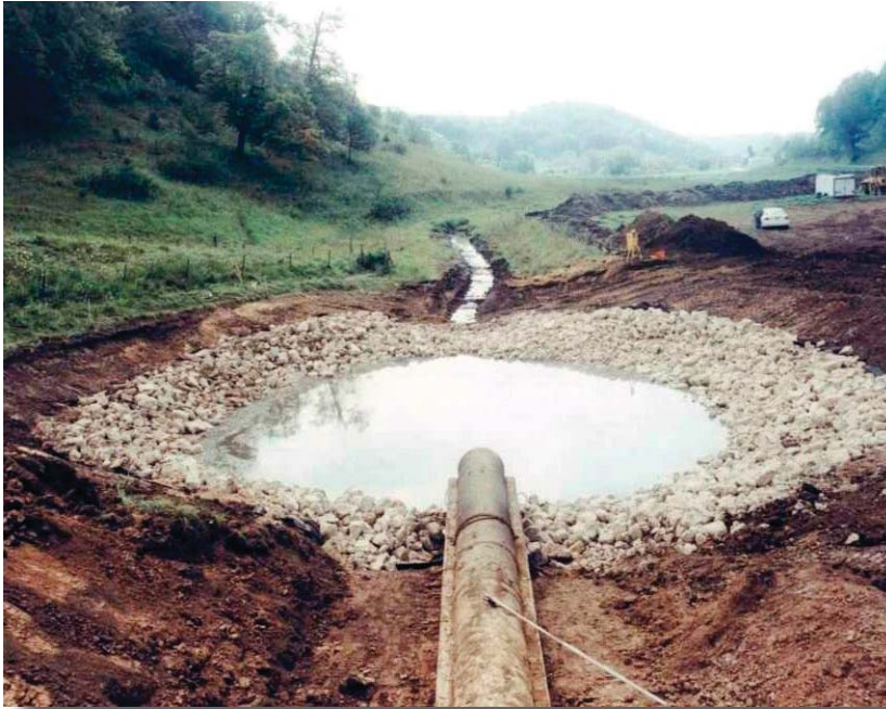
Rehabilitated plunge pool.
