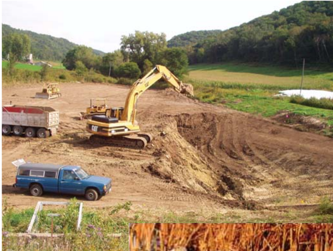
Removal of sediment from Alma Mill Creek structure No. 3.
