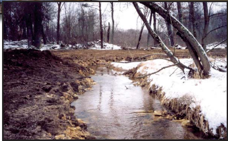
Lyndon Creek after streambank restoration completed.
