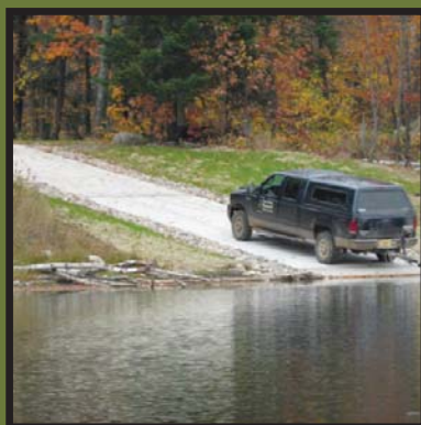
Improved boat landing after construction
