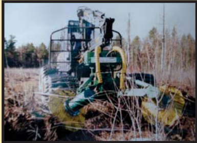
Preparing the site
