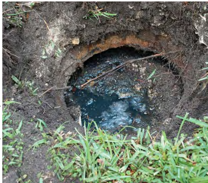
View inside a septic system with clogged drainage.
