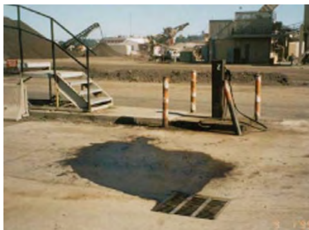
Fuel spills flowing into drains at refueling stations like this one are a common source of ground water contamination.
