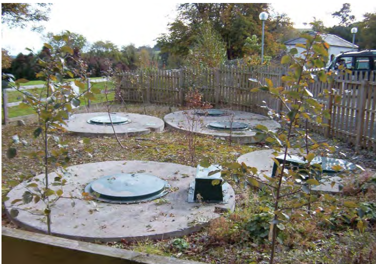
Figure 4. "Community" leaching fields serving multiple single-family homes, with their open space, environmental and aesthetic benefits, are now fully approvable in most states. This plat shows a proposed community leaching field in Connecticut that will be assessed by the Department of Environmental Protection for approval of the hydraulics of the proposed system, the treatment of nitrogen and pathogens, and the mixing of treated wastewater into the area's ground water system. The location of the proposed system's leaching fields, affected soils, the supporting ground water system, and adjacent areas are factors that will influence the design and feasibility of the system.
