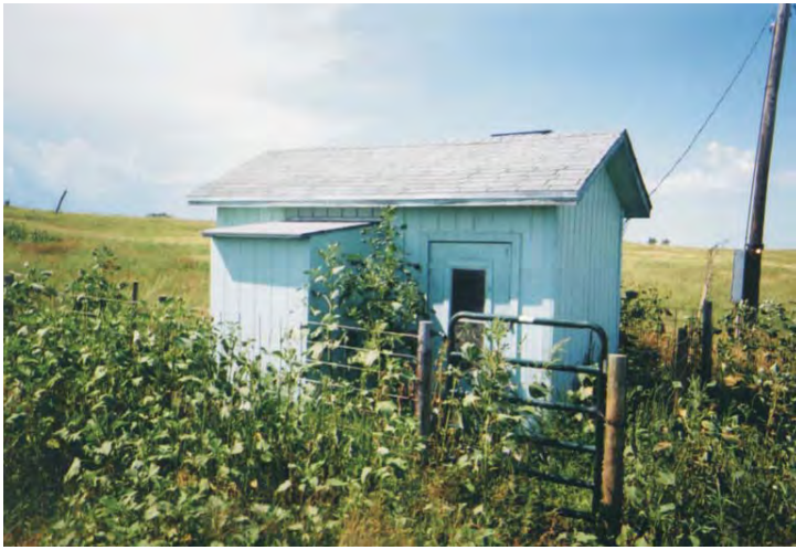
A well house for a municipal well in Tripp County, South Dakota.
