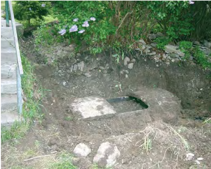
A malfunctioning septic tank that is being cleaned out and repaired.
