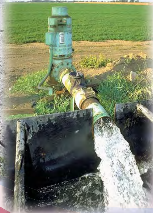
Left: Ground water pumping in the Arizona desert has caused the land to subside in some basins.
