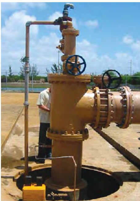
Treated municipal wastewater is pumped more than 3,000 feet deep underground through a Class I injection well in South Florida.
