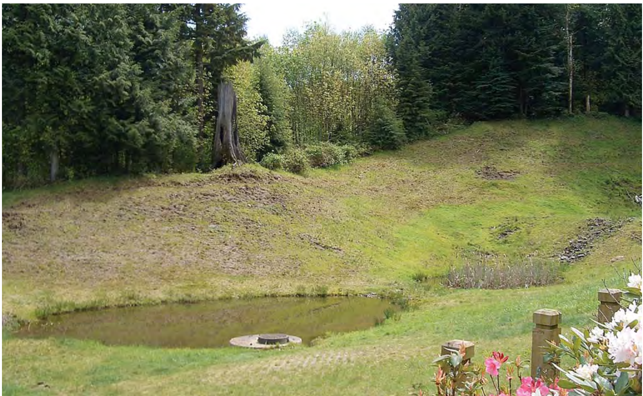
A system of stormwater infiltration ponds in the Uplands neighborhood of North Bend, Washington.
