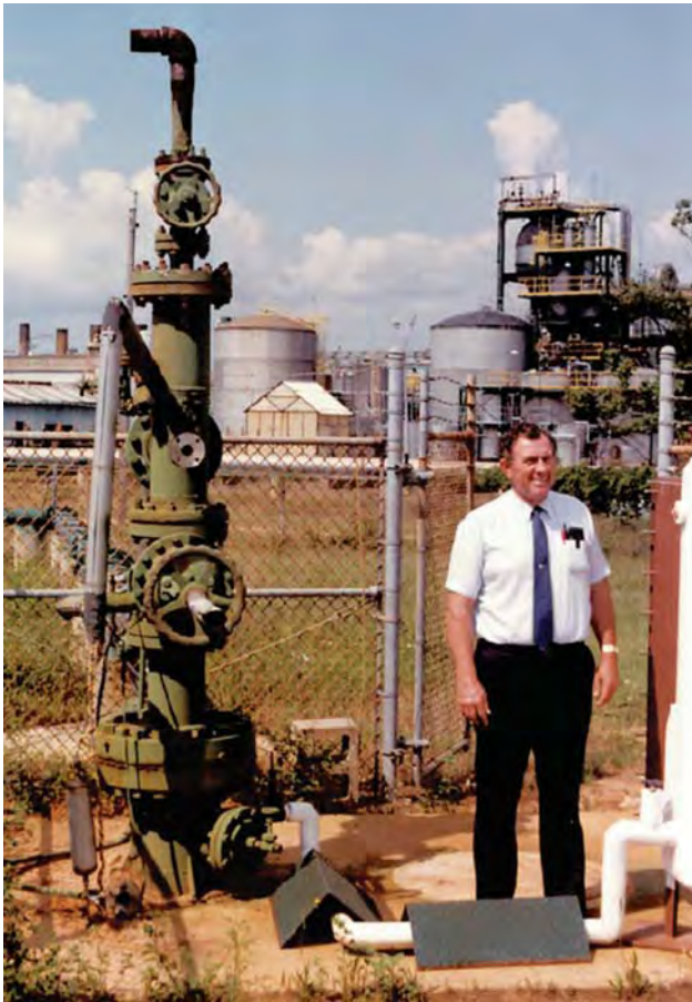
Neale Sharitz at an industrial primary injection wellhead that Sterling Fibers, Inc. constructed in 1971 in Milton, Florida. This wellhead configuration is typical of a Class I disposal well at an industrial facility.
