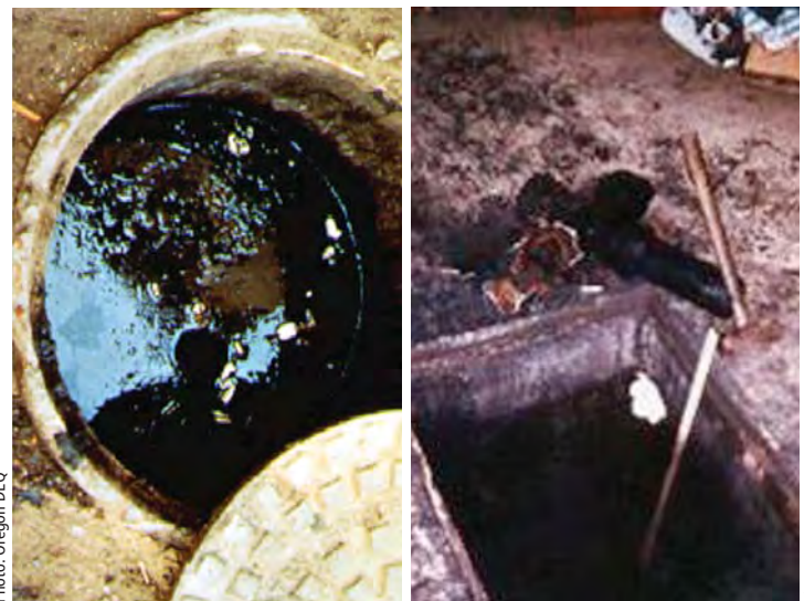
Floor drains and open pits such as these pose a substantial threat to ground water.
