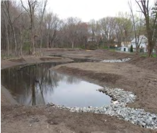
New Stream Channel
