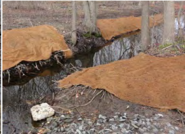
Channel at Oxbow #3 with erosion control matting on banks
