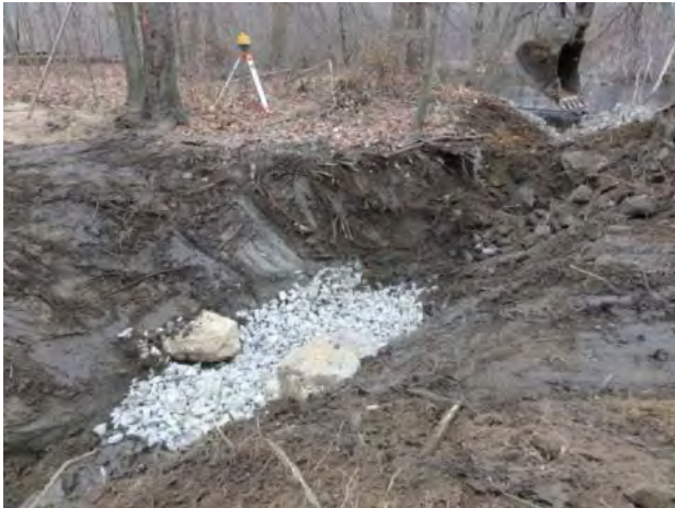
Re-establishing connection to Pawtuxet River at Oxbow #3
