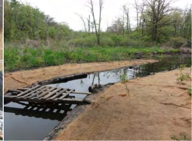
Channel at Oxbow #2 with erosion control matting and plantings
