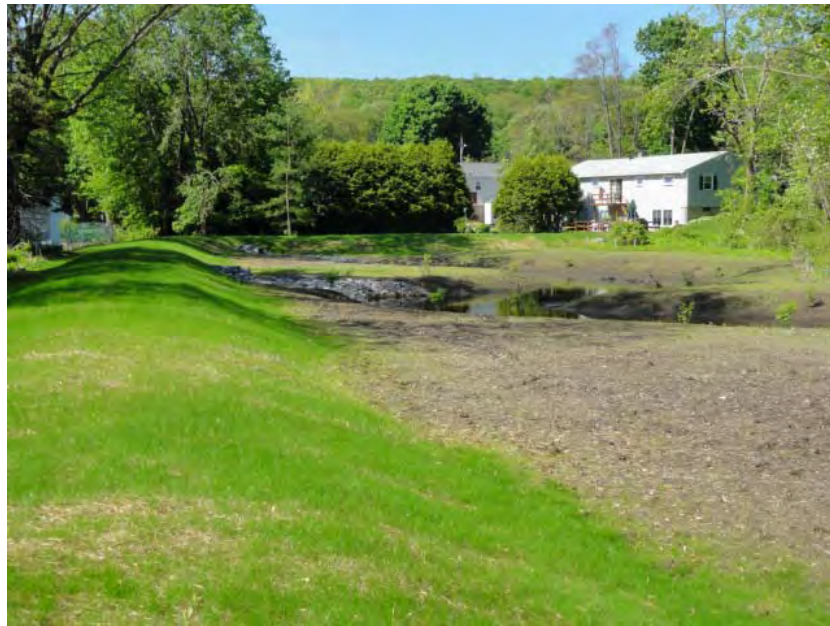
New Earthen Berm
