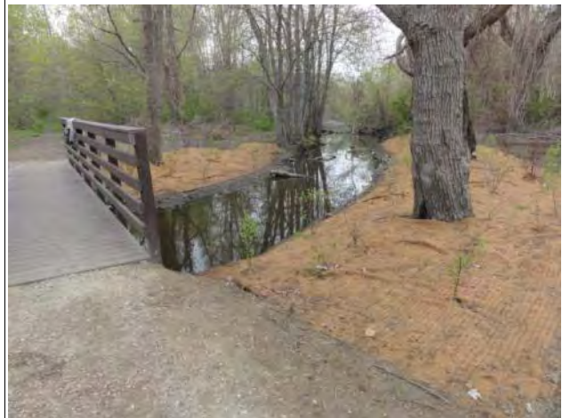
Bridge and channel at Oxbow #1 post-construction
