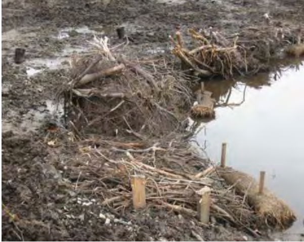
Brush mattresses/Root wads along new stream bank
