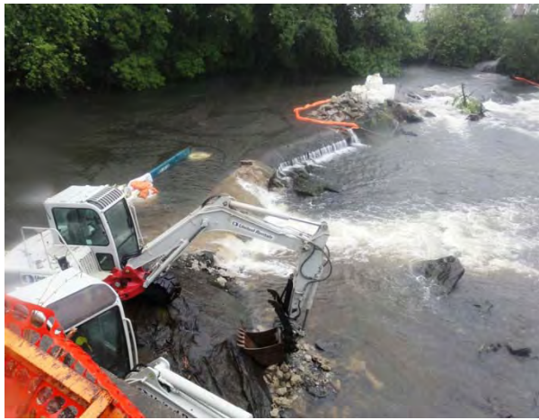
The removal of the spillway required excavators fitted with hydraulic hammers to break up 150 feet of concrete (left) and Pawtuxet Falls after the dam removal (right).
