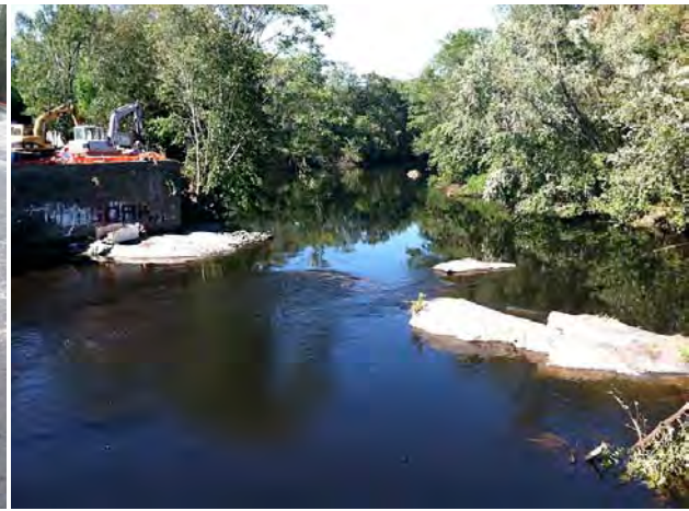
The removal of the spillway required excavators fitted with hydraulic hammers to break up 150 feet of concrete (left) and Pawtuxet Falls after the dam removal (right).
