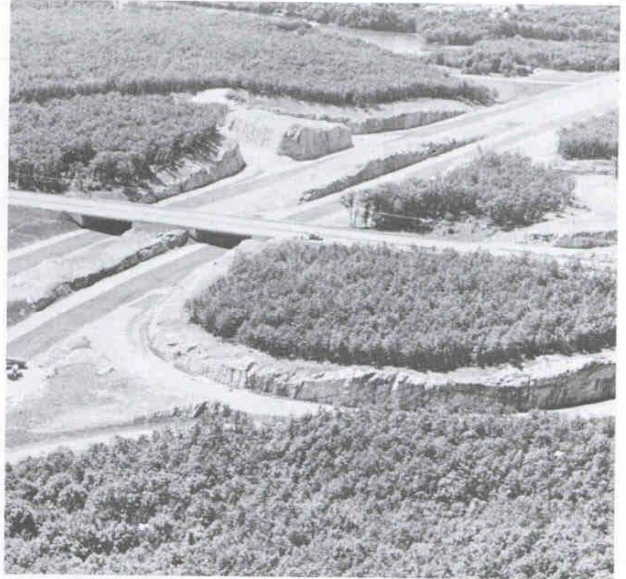
Large areas of land are required for interstate highways and, where bedrock is near the surface, construction costs are high.
