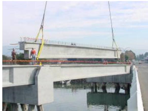
Replacement of ISC Alameda Bridge (January 2002)
