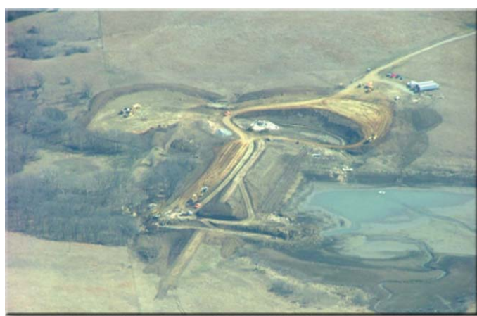
Rehabilitation construction on Double Creek site 5, in Washington County.
