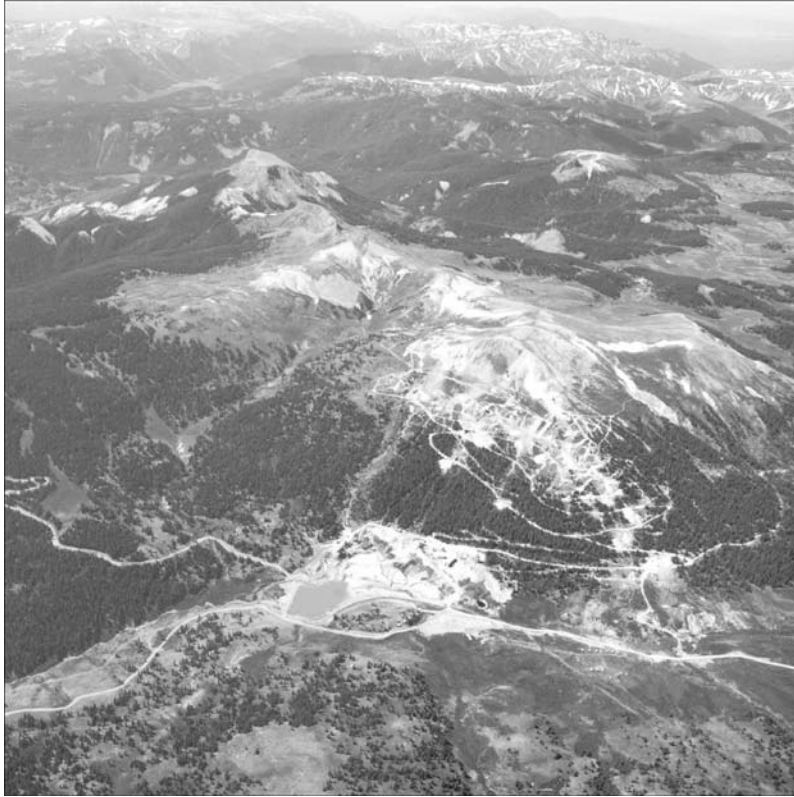
Figure 2-34. Photo of Summitville Site in 1980 Prior to SCMCI Operations
