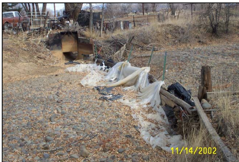
Figure 2-106. Dam Constructed of Marginal Materials – Cristobal Rivera Ditch
