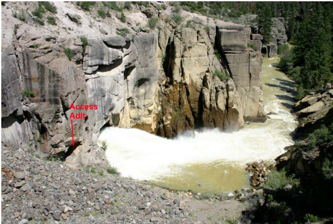
Figure 2–85. Terrace Reservoir Discharge Portal and Access Tunnel
