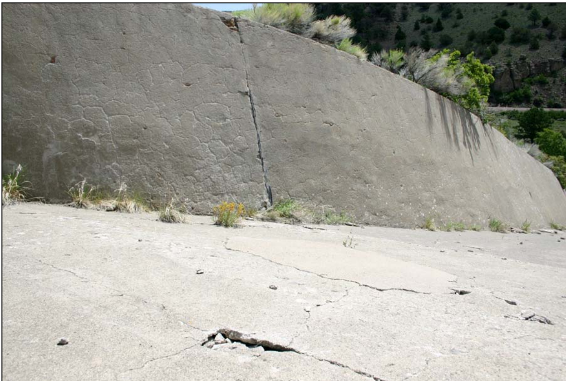
Figure 2-84. Condition of Terrace Reservoir Spillway Concrete and Masonry Approach Walls
