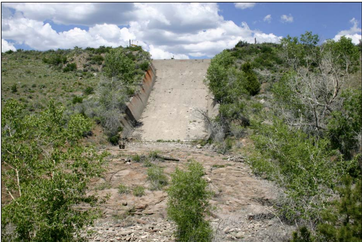
Figure 2–82. Terrace Reservoir Spillway from Downstream
