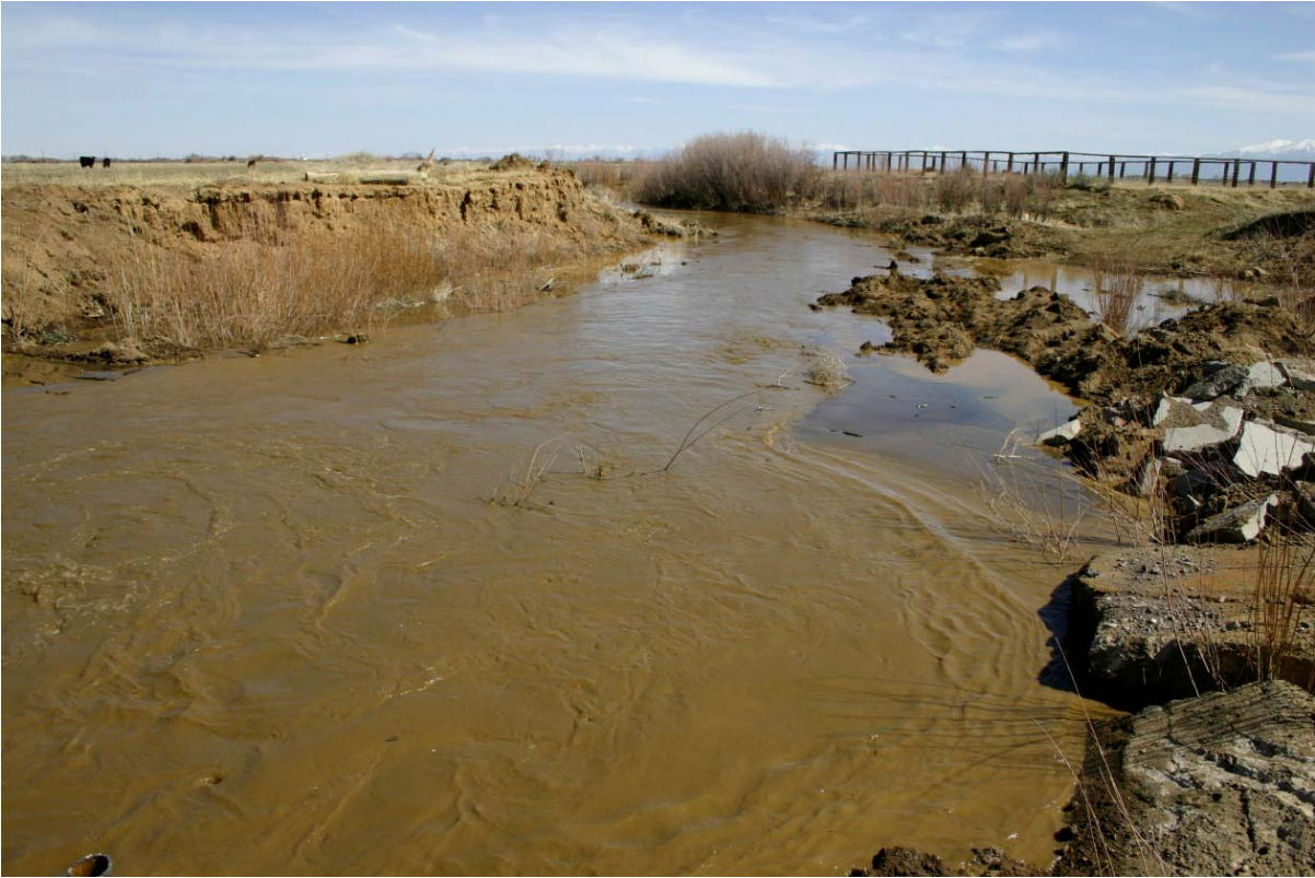
Figure 2–107. Photo of Terrace Sediments Flushed into Head Overflow #5 Ditch
