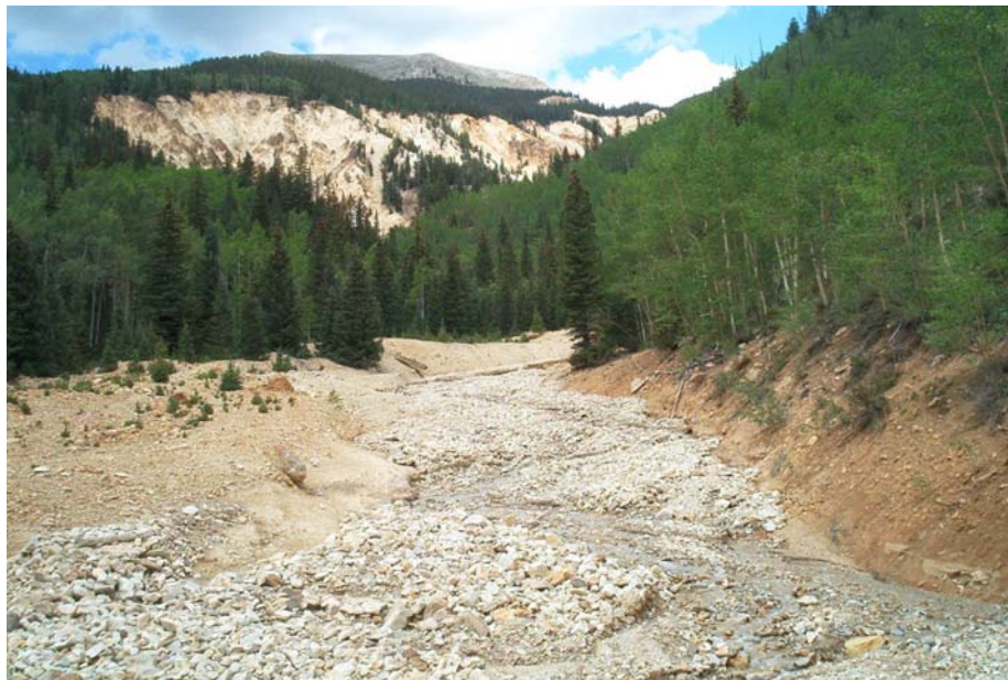
Figure 2-93. Photo of Alum Creek Channel Showing High Sediment Load
