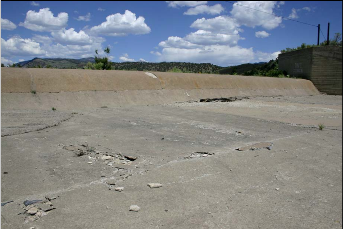
Figure 2-83. Terrace Reservoir South Abutment and Spillway from Downstream
