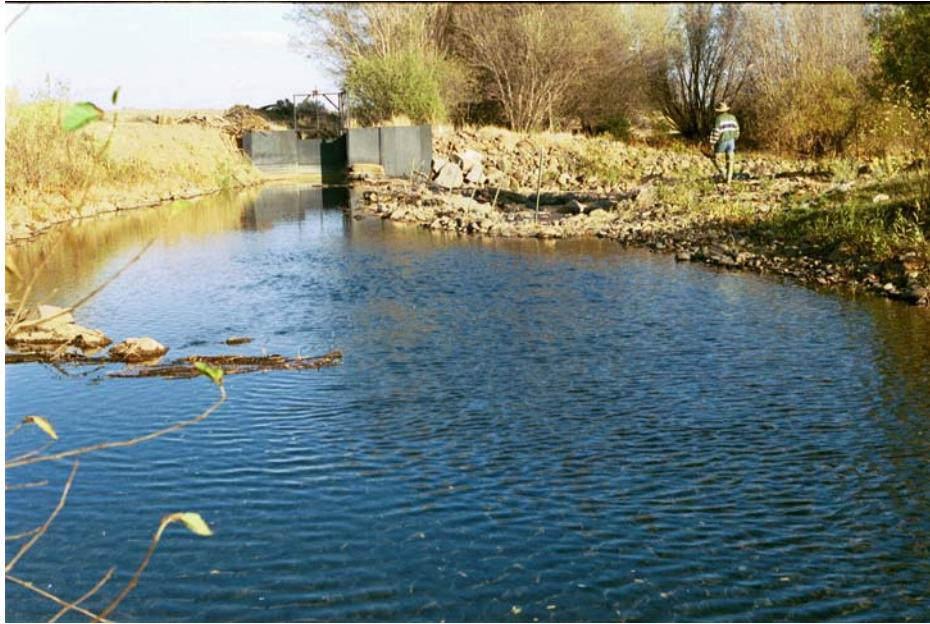
Figure 2-13. Photo Above Irrigation Diversion (photo by Alan Miller)
