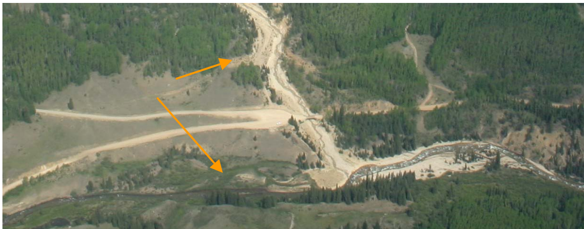
Figure 3-19. Aerial Photo of Alum Creek Confluence
