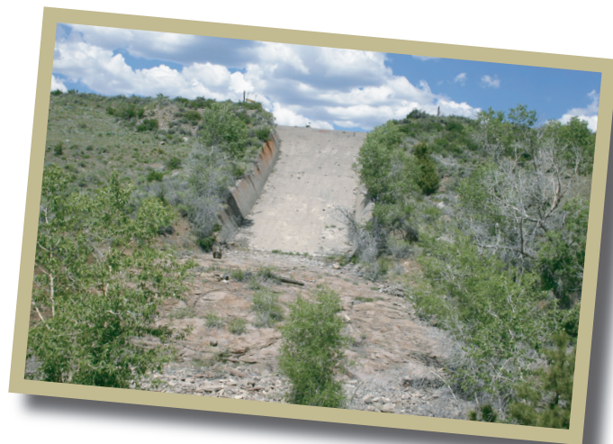
Figure ES-7. Terrace Reservoir Spillway from Downstream
