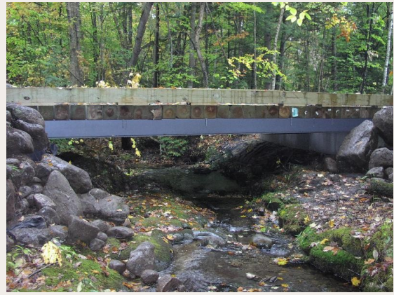
Bridge Stream Crossing Installed (After)
