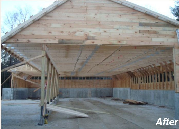
Muddy heavy use area replaced with a roofed concrete manure storage and heavy use area.
