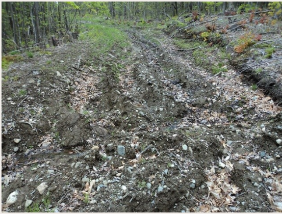
Access Road (Before)
