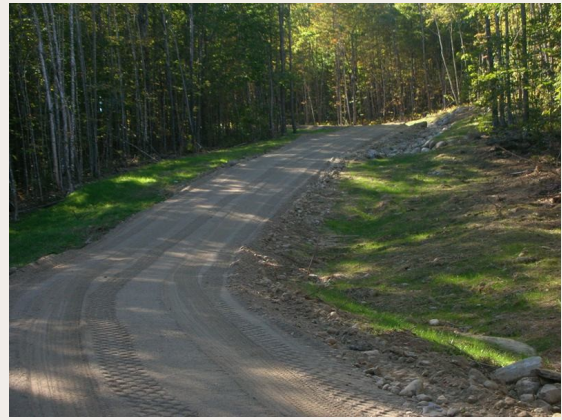
Access Road (After)
