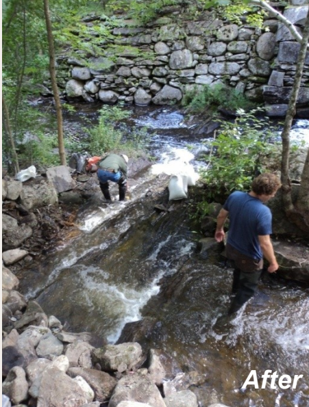
Pullen Mill – A pool and weir fish passage were installed.
