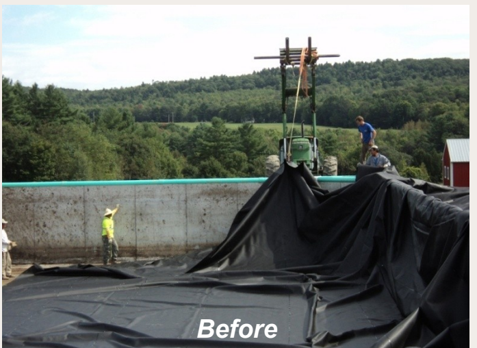
Methane digester project on organic dairy farm. Installation of the cover over the manure pit will be used to collect methane for digestion.
