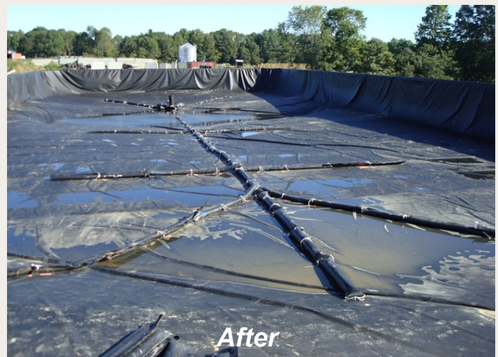
Methane digester project on organic dairy farm. Installation of the cover over the manure pit will be used to collect methane for digestion.
