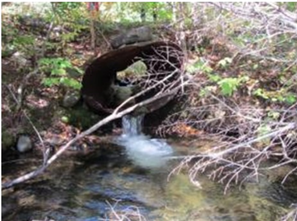
The above photos show the before and after construction of the first culvert that was removed on a tributary to Mountain Brook in 2012. The pre-existing culvert was a 4-foot round boiler pipe, it was replaced with bridge abutments with a 14-foot span.
