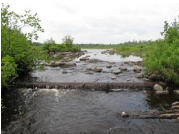
The above photos show the before and after deconstruction of a remnant log drive dam on Roaring Brook.
