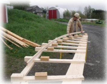
Sunny Stutzman working on the framing for the CIG high tunnel.
