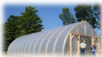
The finished CIG high tunnel at Stutzman's Farm in Sangerville.
