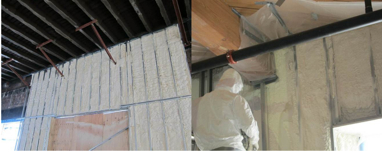
Figure 8. Various retrofit installations of interior spray foam insulation on mass masonry
