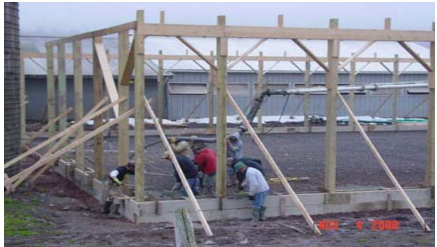
Covered barnyard during construction to reduce pollution and improve quality.
