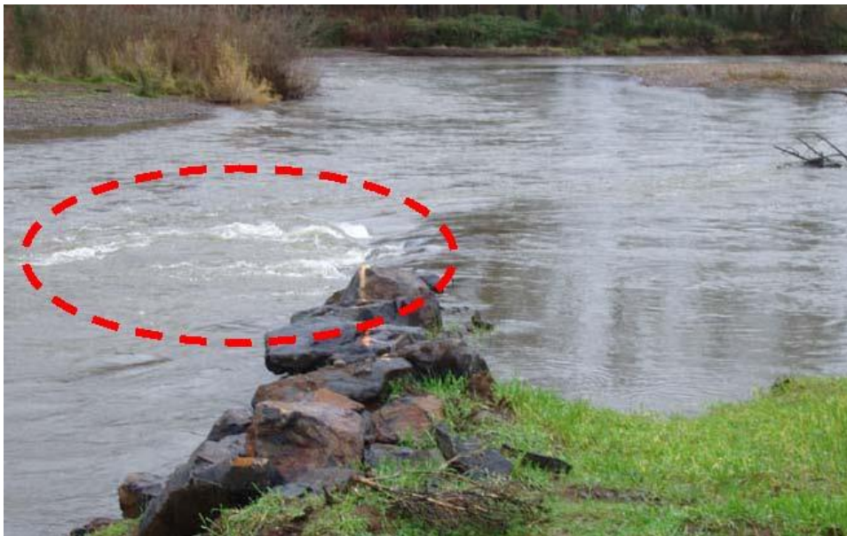
Figure 5—Turbulent zone at intersection of cross structure flow and contraction accelerated flow at 75 percent bankfull discharge
