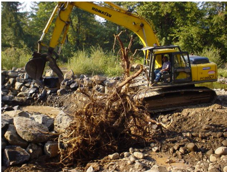
Figure 9–Large wood placement within barb section
