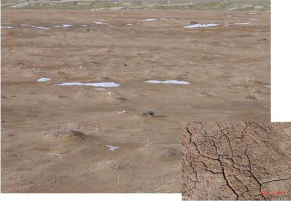
Figure A-3. Landfill Cover Located on the Navajo Reservation that experienced significant Wind Erosion
