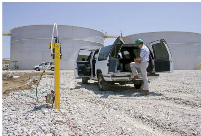
Figure 3-4: Example of a Groundwater Monitoring Well
