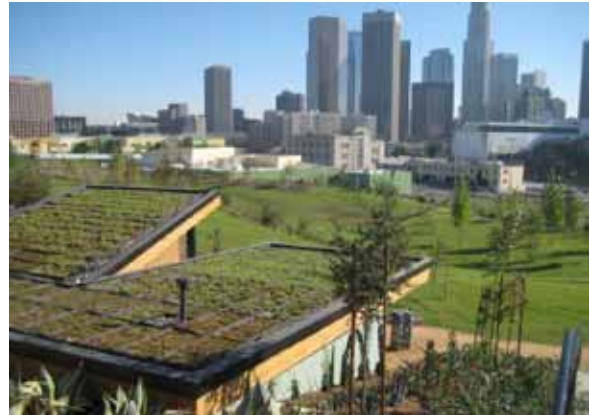
Green roof in Vista Hermosa Park, Santa Monica Mountains Conservancy, Los Angeles / CREDIT: Ken Weston and Reza Iranpour/ City of Los Angeles
