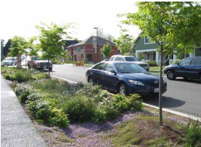
Drainage swale as part of Seattle’s SEA (Street Edge Alternatives) Project / CREDIT: EPA/ Abby Hall
