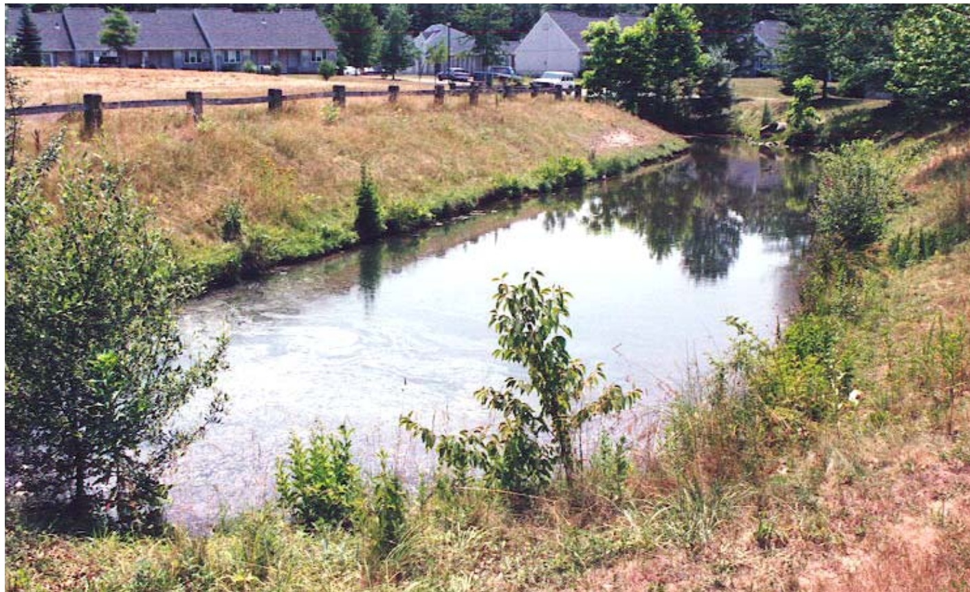
Fig. #2 Storm water pond Photo Credit: Tom Ladny, NRCS
