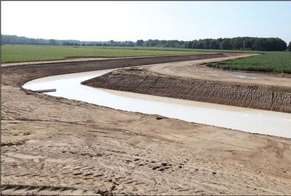
A tailwater recovery system catches runoff water from fields to be pumped into an irrigation reservoir for storage.
