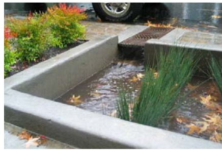
Above, the same planter during a rain event, where it is easy to see how much water can be captured and diverted from conventional underground pipes. photo: Kevin Robert Perry
