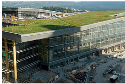
Vancouver's Convention and Exhibition Centre will include a green roof, energy efficient systems, and greywater treatment. photo: www.roofculture.com/gallery/vancouver/
