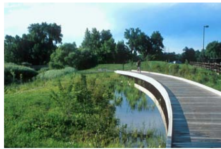
This constructed wetland near Denver, CO manages all of the surface runoff from an adjacent parking lot. photo: www.werf.org/livablecommunities
