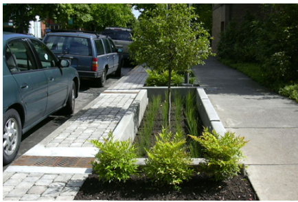
Stormwater infiltration planters in use in Portland, Oregon at Southwest 12th Avenue Green Street. The above image shows a newly installed planter in dry conditions. photo: Kevin Robert Perry
