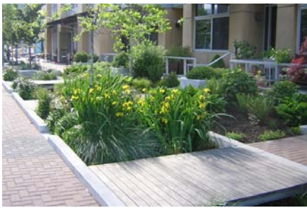
Permeable pavement and swales are part of the stormwater management plan for Portland's South Waterfront. Lush plantings are possible without watering maintenance. photo: Nevue Ngan Associates
