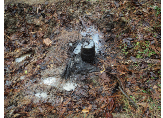
Leaking well head/USFWS
