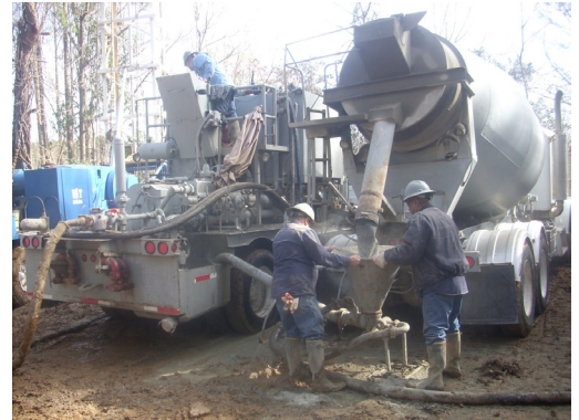
650 sacks of concrete were required to properly plug the well/USFWS
