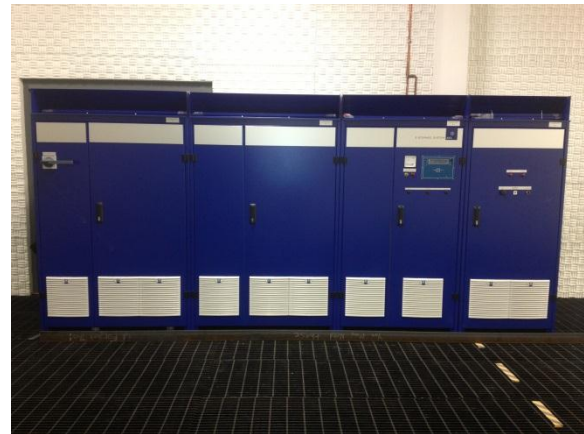
Figure VI-53: AVL e-storage unit installed at ORNL VSI laboratory.
