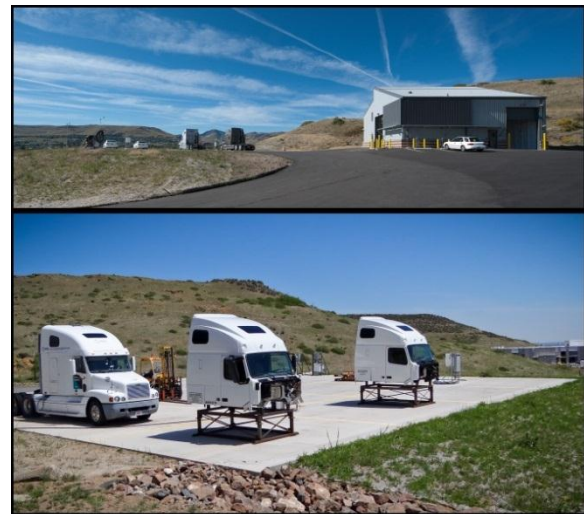
Figure V-152: NREL's Vehicle Testing and Integration Facility.
