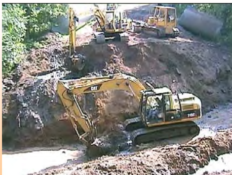
Excavation to a Fish Friendly Elevation
