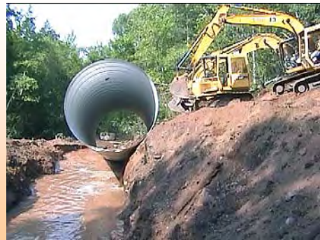
Dropping in the First 40 Foot Section
