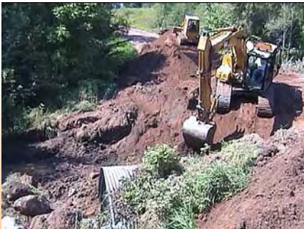
Removal of Old Pipe and Creation of Bypass Channel
