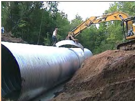
Banding Together the 2 Sections
