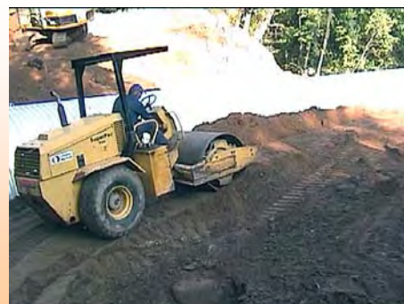
Compaction of Clean Fill Around Pipe
