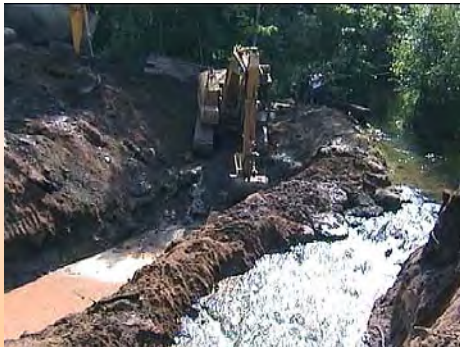
Stream Bypass Channel
