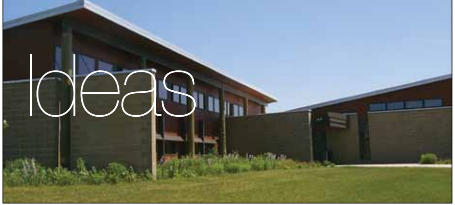
IAMU's office structure is an award-winning example of sustainable design. Along with an adjacent 11-acre safety & training field, it serves the association's member utilities in many ways.
