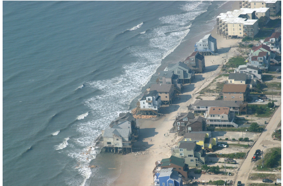
North Topsail Beach, North Carolina after Hurricane Ophelia.
